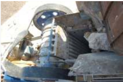
Crusher Jaw Plates in operation
